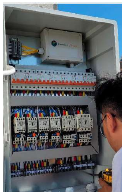
Figure 6. Inside photo of controller FARMEXT.
